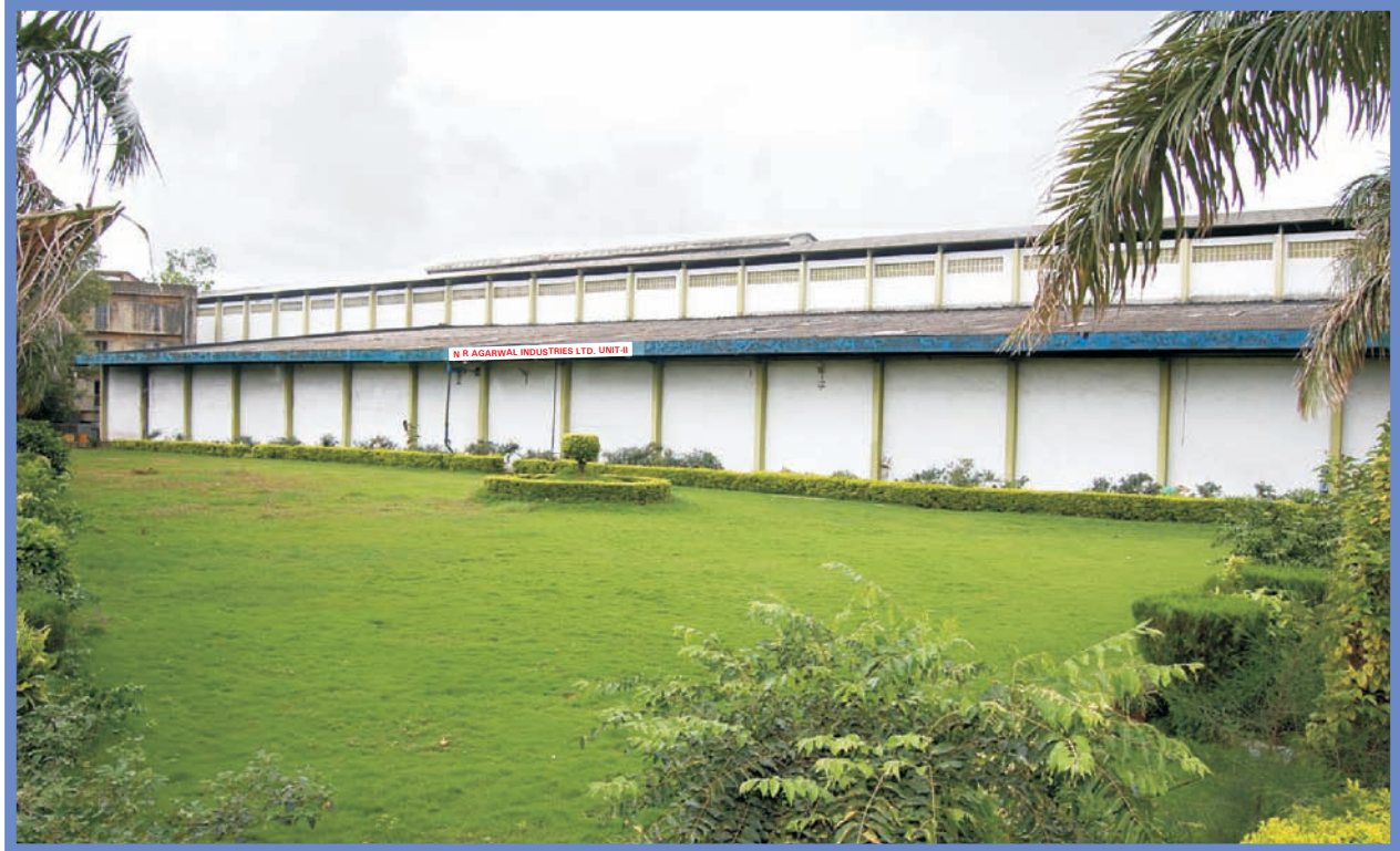
VAPI FACTORY (UNIT II)
